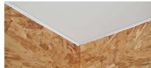
Image B08 - corner assembly - with textile
