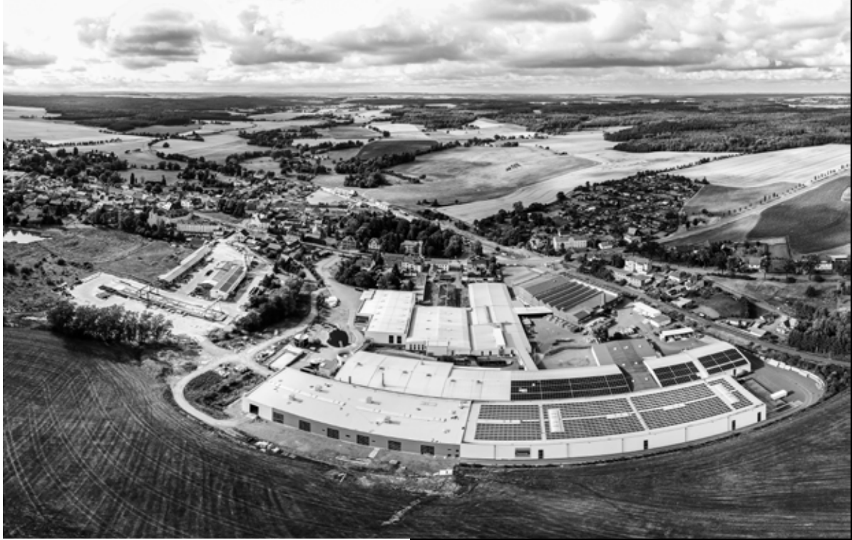
Location: Mühltröf PONGS Technical Textiles
