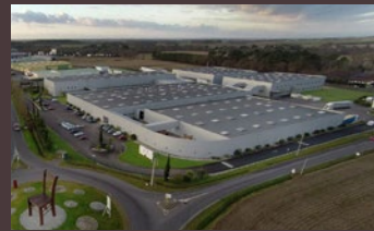
HAGETMAU FACTORY BUILDING 24 000 m 2
